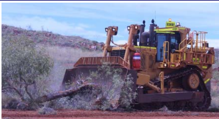
Figure 1 : AJM has begun on-site project construction
