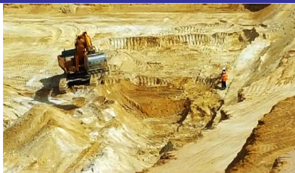
Figure 5b : over-burden cleared
