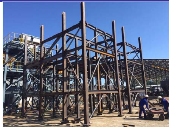
Figure 3b : Off-site trial erection of plant
