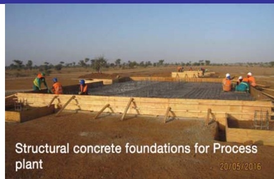
Figure 4b : Structural foundations
