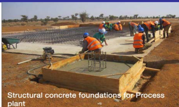
Figure 4a : Foundations for processing plant
