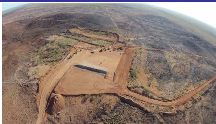
Figure 1 : Tabba Tabba : plant site prepared
