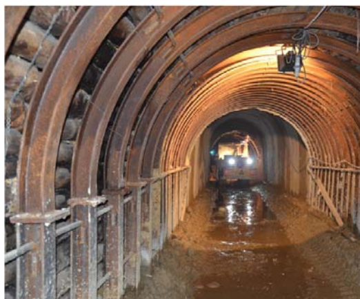
Figure 6a : refurbishing access to Gorno
