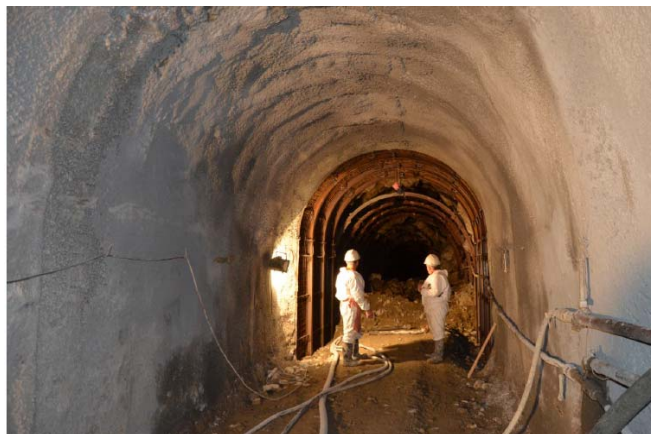
Figure 6b : refurbishing access to Gorno
